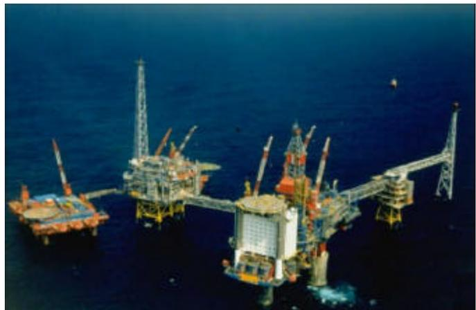
Figure 1: The Sleipner natural gas drilling platform. CO<sub>2</sub> is separated from the gas and reinjected to a saline aquifer. ([www.statoil.com](http://www.statoil.com))
